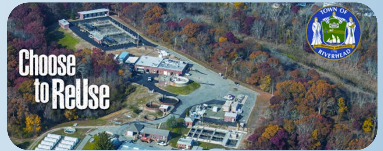
Riverhead STP (photo illustration by H2M Architects & Engineers)
